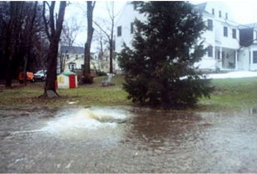
SSOs, which contribute to flooding, will be eliminated throughout the District's member communities.
