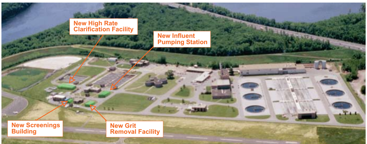
A new influent pumping station, and new grit removal and wet weather treatment facilities will help handle increased flow to the Hartford WPCF.
