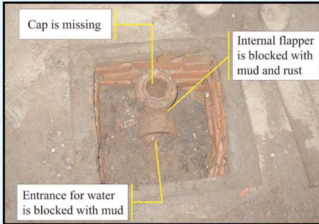
Backwater Valve allowing waste waters to flow to the sewers.
